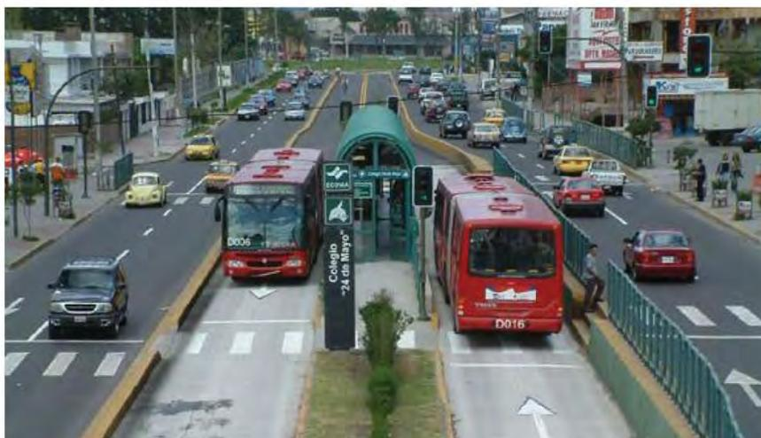
Fig 75 - Alternative 2 - Median-Running Bus (BRT)
