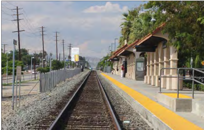
Northbound rails at the Sylmar/San Fernando MetroLink Station
